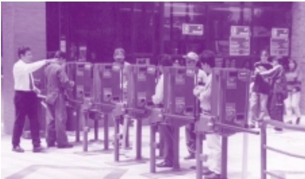
Quito's BRT features a pre-boarding fare card system (courtesy Lloyd Wright, ITDP).
