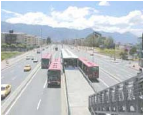
Four-lane roadway. Inner lanes dedicated to station enables high-speed bypass (Source: Transmilenio S.A.)
