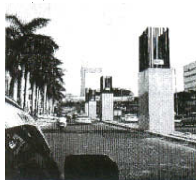
Photo 5. Monorail under-constructed at Rasuna Street 10)
