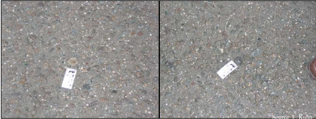
Figure 77: A magnet protected by an elastomer, above the metro ticket
