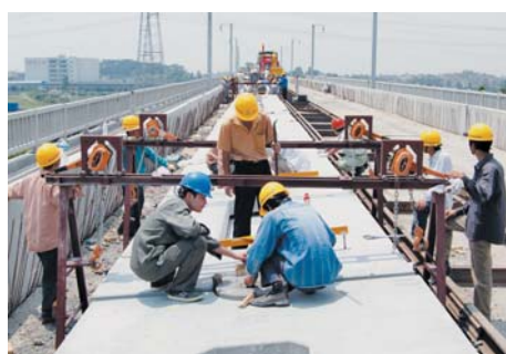
Slab track technology transfer on Guangzhou test line (China)
