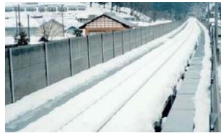
Snow-melting warm water panel equipment (Hokuhoku Line)
