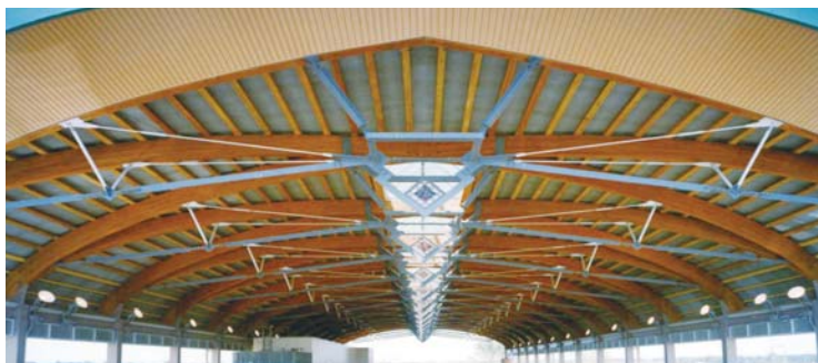
Miraidaira Station, Tsukuba Express [Japanese larch from Hokkaido is used for the beams of the large roof]
