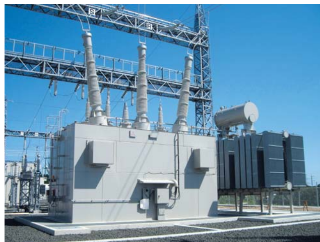
Roof delta connected transformer, Shin-Shichinohe substation, Tohoku Shinkansen
