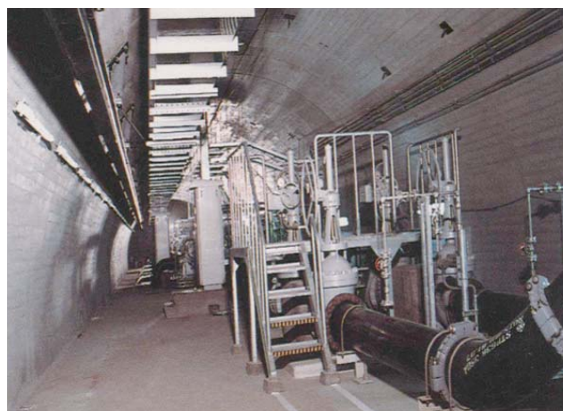
Pump chamber pumping out seepage water
