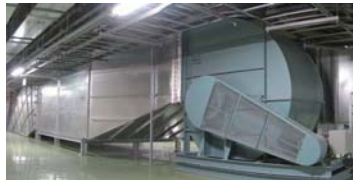
Ventilator room for tunnel (Minatomirai Line)
