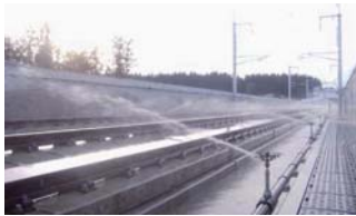
Snow-melting sprinklers (Tohoku Shinkansen)
