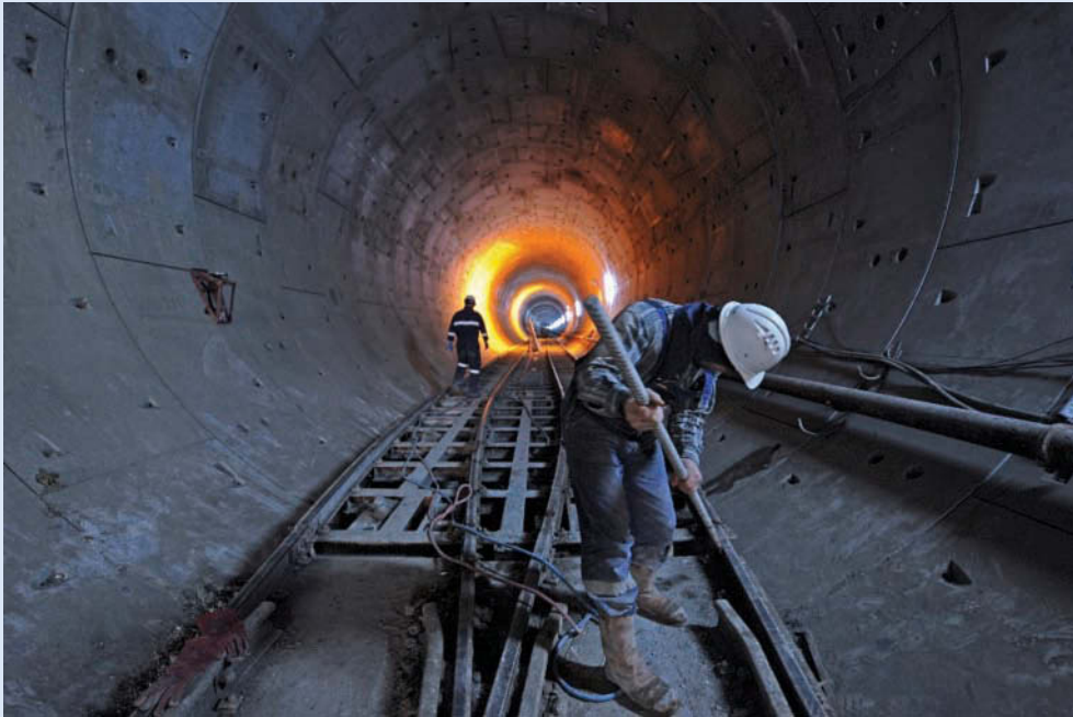
IMAGE B17.5.1. Workers in the Earthquake-Resilient Marmaray Tunnel: Istanbul, Turkey
