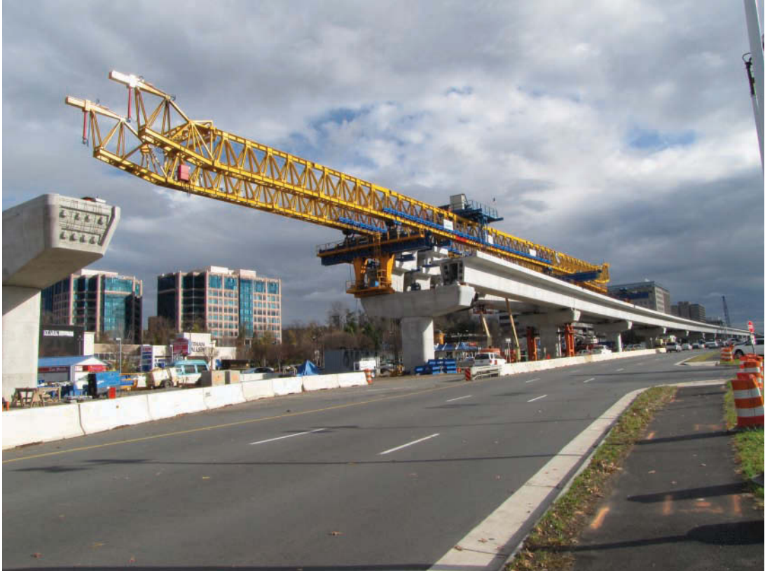
IMAGE 11.2. Building the Deck Span across Vertical Supports: Silver Line, Washington, DC
