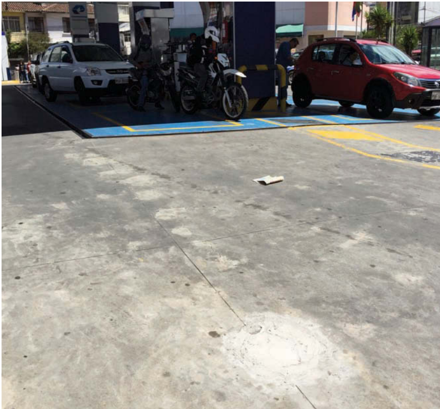
IMAGE 15.2. Pavement Perforation to Test Soil and Groundwater Contamination at Gas Station along Rail Right-of-Way: Quito, Ecuador
