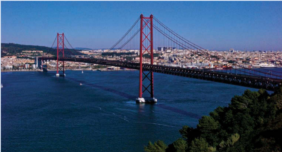
IMAGE B6.1.1. Highway and Rail Bridge across the Tagus River, Portugal
