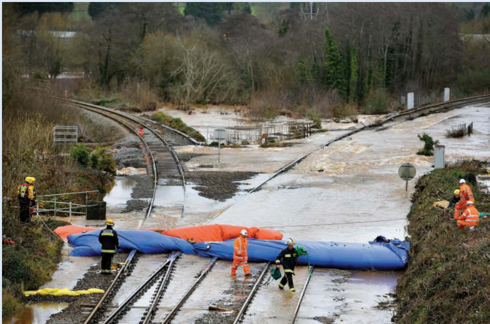
IMAGE B17.3.1. Railway Engineers and Fire and Rescue Service Personnel Watch Over Inflatable Dams Protecting the Tracks at Cowley Bridge Junction
