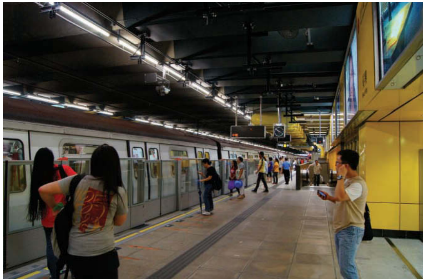
IMAGE 5.1. Half-Height Platform Screen (or Edge) Doors: Kwai Hing Station, Hong Kong MTR, Hong Kong SAR, China
