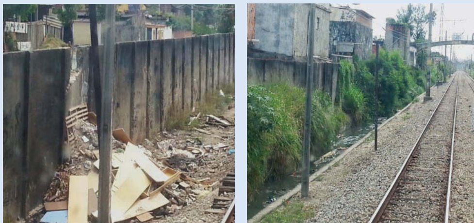
IMAGE B15.6.1. Illegal Solid ( left ) and Liquid ( right ) Waste in Rail Right-of-Way
