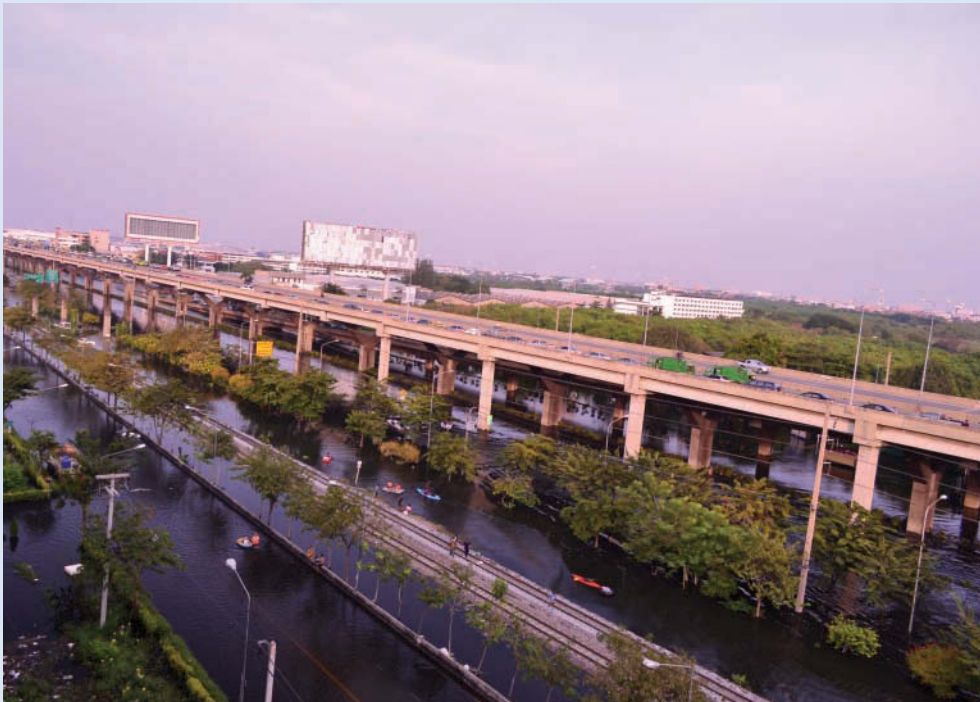
IMAGE B17.2.1. Skytrain Track Elevated above Monsoon Flood Levels, Bangkok, Thailand
