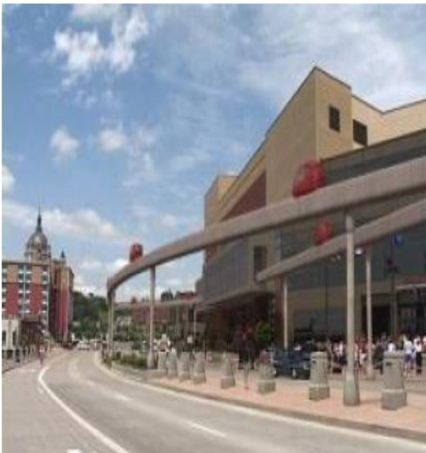
Figure 6: PRT system, with off line station inside building Source: Anderson, J.E., 2007 and Skyweb homepage, n.d.
