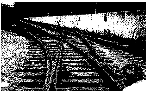
Figure 6.5.2 Tongue Switch and Mate—Non-embedded 149 RE 7A Rail
