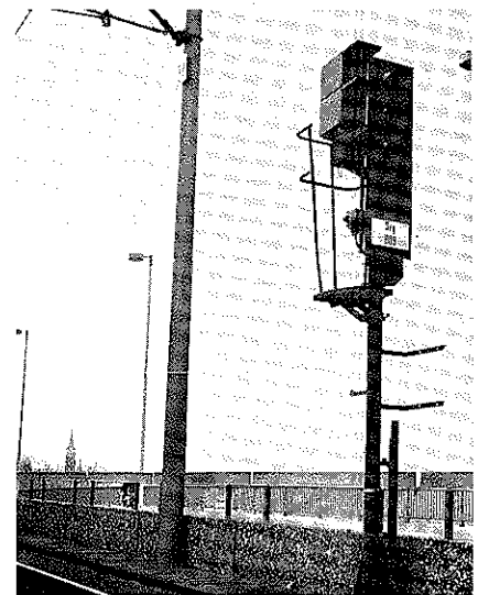
Fig. 5: Signal with platform, safety barrier and mounting for signal telephone set on the Deutzer Brücke on the Rhine
