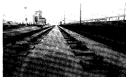
Fig. 6: The track towards Deutz (on right) already in service on the new Deutzer Brücke, the track towards Cologne (centre) in construction. It adjoins the old track towards Cologne (left of white line) which is still in operation on the old steel bridge (mid-October 1979)
