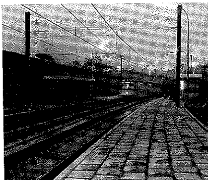
Fig. 7: The first German double-track section on a bearing slab with earth foundation, some 1200 m of track at Cologne-Höhenhaus, early morning on 31st October, 1973, two months after the start of the construction
