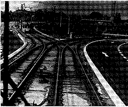
Fig. 4: Junction of the Gürtel section (left) with the western ramp of the Mülheimer Brücke, with a switching section at 500 m radius (1974)
