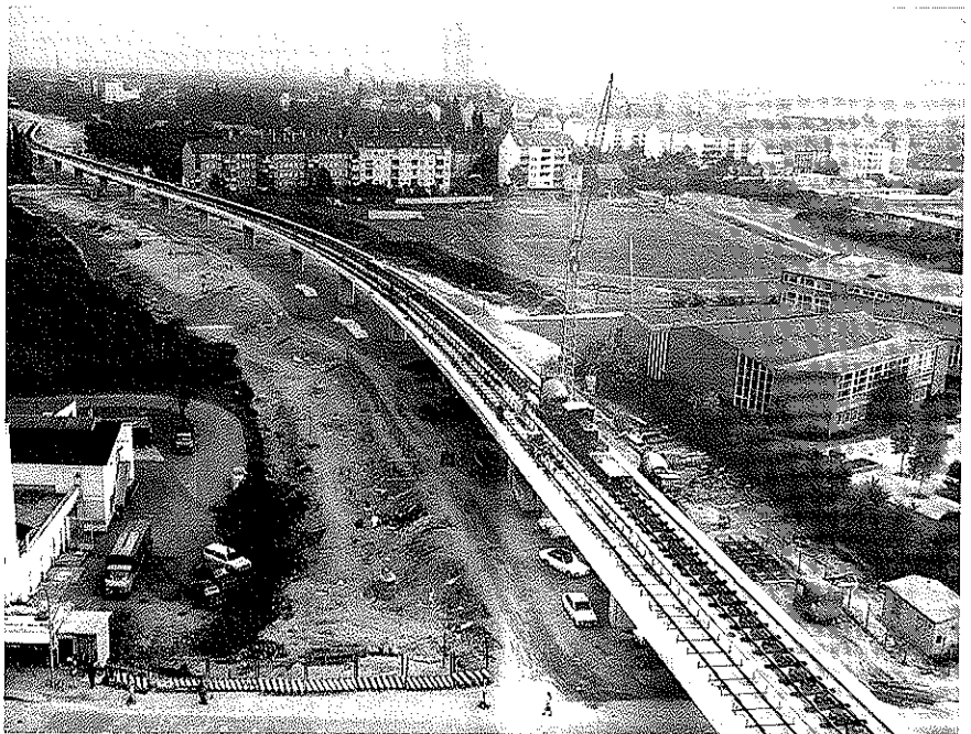
Fig. 6: Elevated rail section in construction (1972). Daily rate of completion: 54 m of track, mobile construction site some 600 m long (with 11 work stages)
