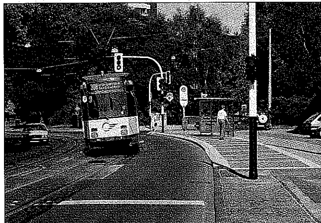
Tram stops are located on the approach to road junctions with traffic lights; passengers using the stops are protected from car traffic by a second set of tram-activated lights (right)
