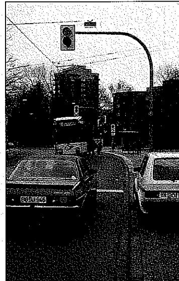
Tram stops are located on the approach to road junctions with traffic lights; passengers using the stops are protected from car traffic by a second set of tram-activated lights (right)
