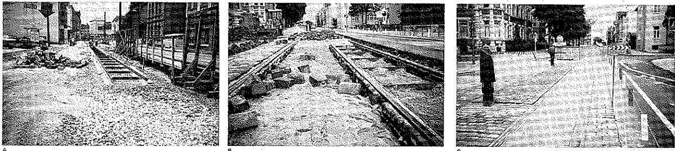
Note: A = preparation of base and assembly, welding, and alignment of track; B = placement of web fillers (hollow clay tile) and sand bed for blocks; and C = placement of blocks and cleaning and sealing of pavement.
