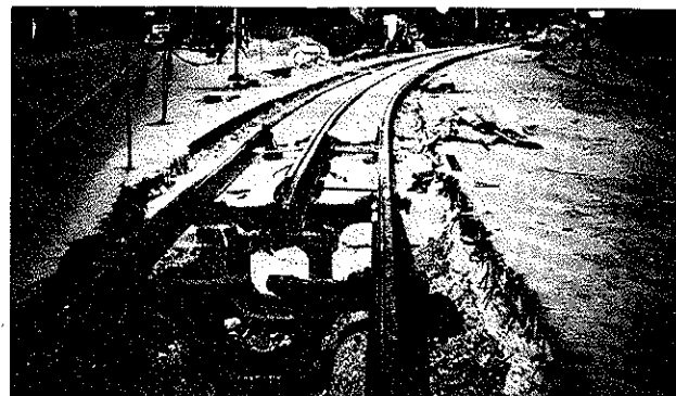
Figure 4. Completely new subsurface installation under construction in London in 1950. (Photo: Julian Thompson)
