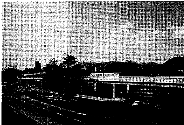
Vancouver's SkyTrain looks like a conventional rail line, but functions without drivers. Opened in 1985, it now carries about 120,000 passengers daily. Courtesy of Bombardier/UTDC
