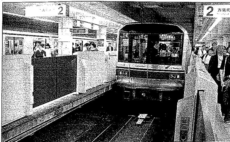
Full platform screen doors were fitted on the ATO-equipped Nambu Line opened in 2000, and Tokyo Metro is testing half-height barriers and gates to improve platform safety on the Marunouchi Line
