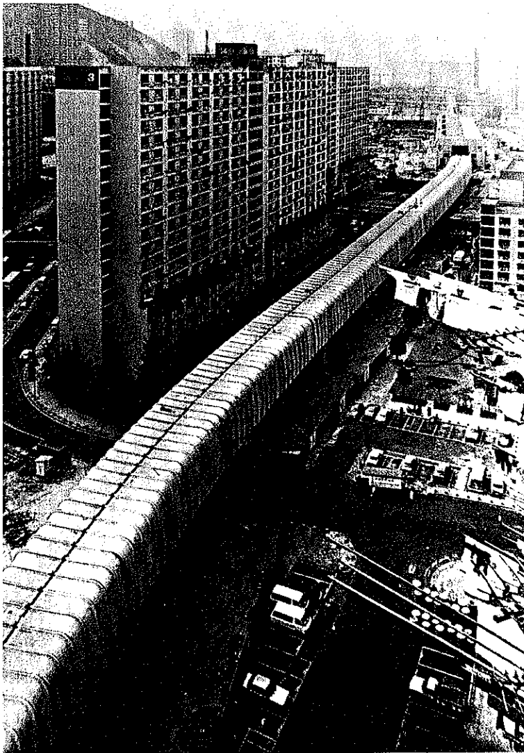
FIG. 16.3. Elevated tunnel to control noise from Mass Transit trains. (Courtesy Mass Transit Railway Corporation, Hong Kong.)
