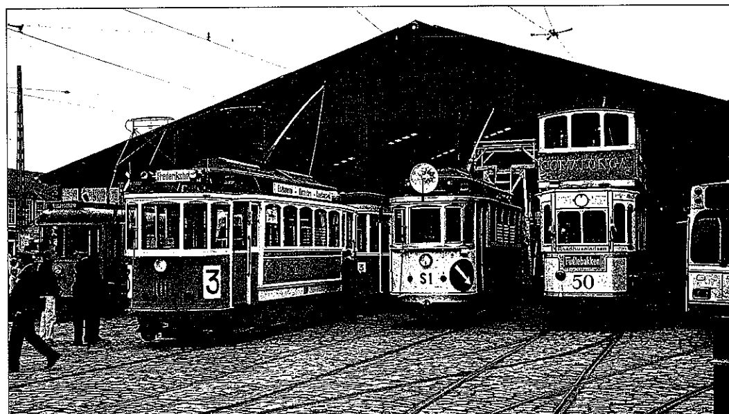
The original museum depot at Skjoldnaesholm features another line-up of København trams, including a former double-decker converted to single deck, a works tram that started life as a double-deck battery tram, and the surviving Frederiksberg double-decker. M. J. Russell
