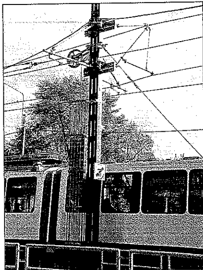
LEFT: Overhead line equipment on Route 41 was upgraded from simple trolley wire to a double-balanced catenary suitable for higher speeds
