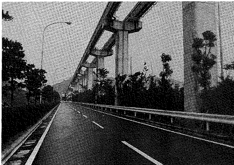
Photo. 8—Pylons erected on median strip (Kita-Kyushu Monorail)
