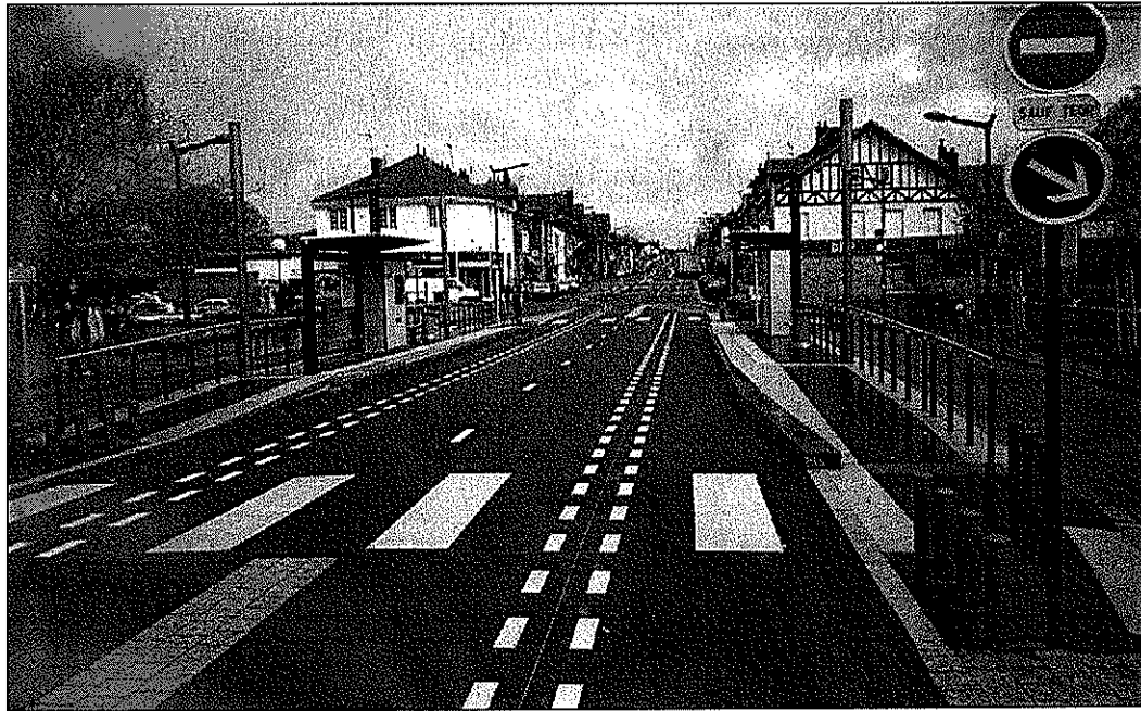
Figure 4: Two-lane Operation at Station
