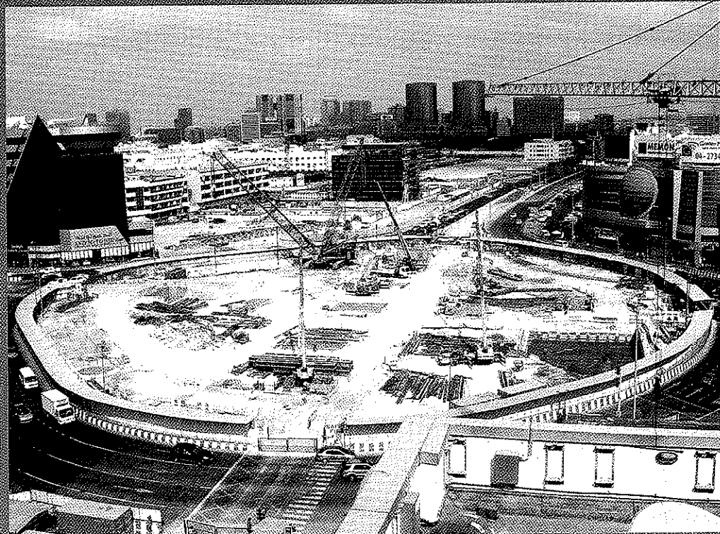
Burjuman Station construction site
