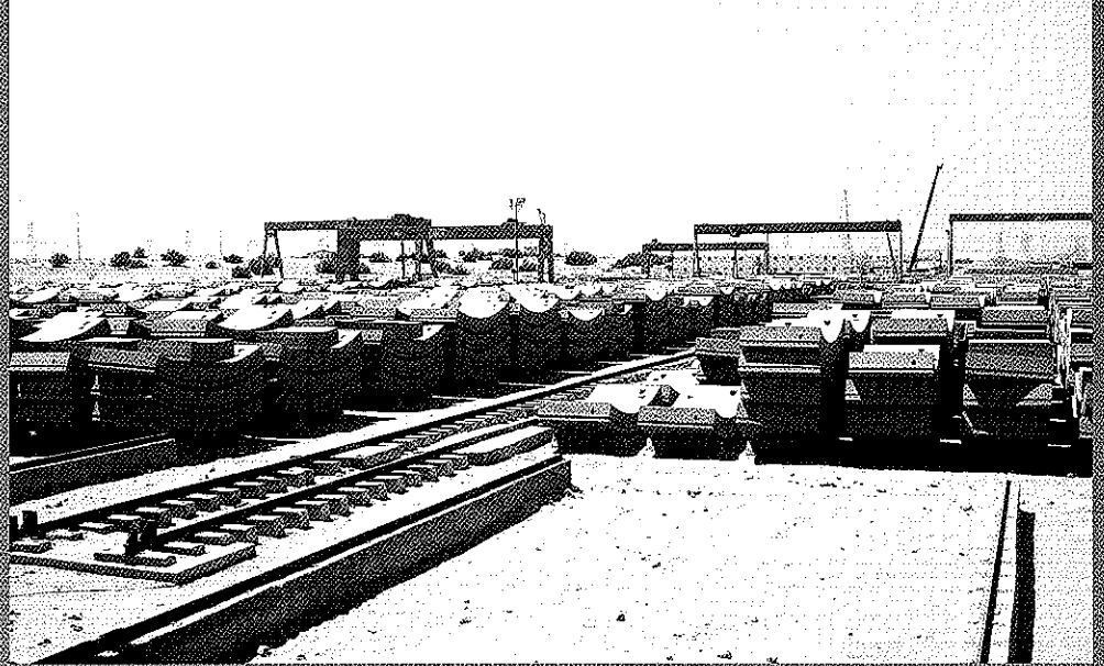
Tunnel Segments Precasting Yard
