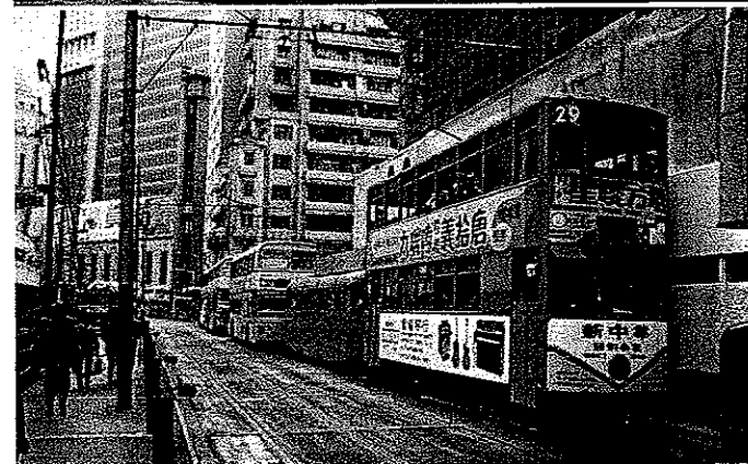
Below: Construction work for the Mass Transit Railway put surface transport into some tight spots in the late 1970s. On a dull December afternoon in 1978, HKT 29 tows a trailer over a plate deck in Des Voeux Road Central, followed by a convoy of buses. The trailers were withdrawn in April 1982.
