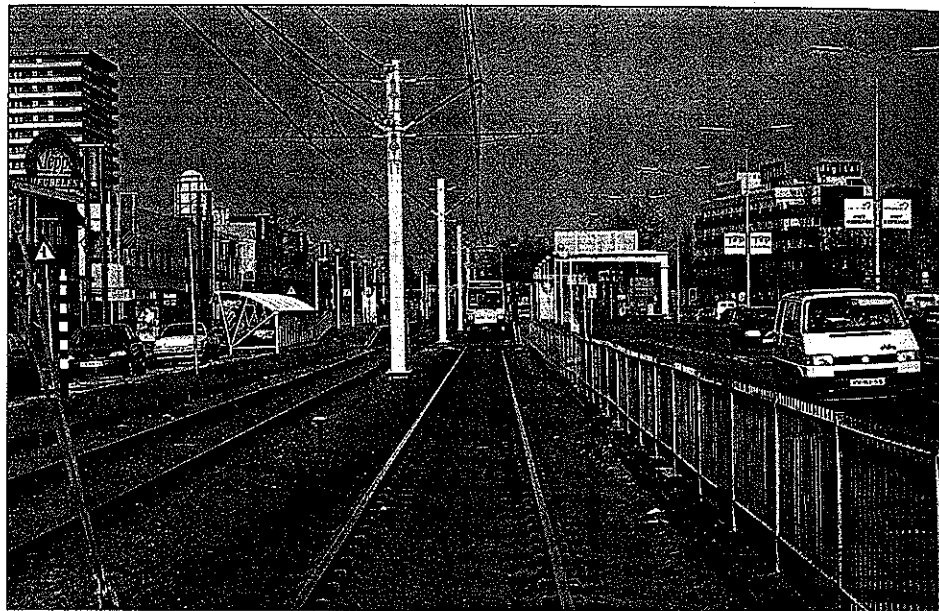
The light rail alignment in the Beneluxaan, south Utrecht, now the most heavily patronised stretch of the system. Note the heavy overhead, built to railway standards. C.J. Wansbeek
