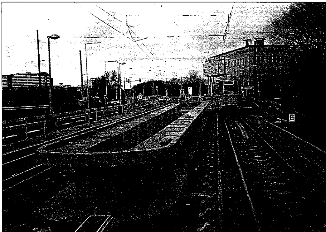
Upgrading work is in full swing on Stuttgart route 15 to Heumaden, where the central platform for standard-gauge Stadtbahn cars is under construction and the metre-gauge GT4 tram will run only until 31 July 1999. G. Wandel
