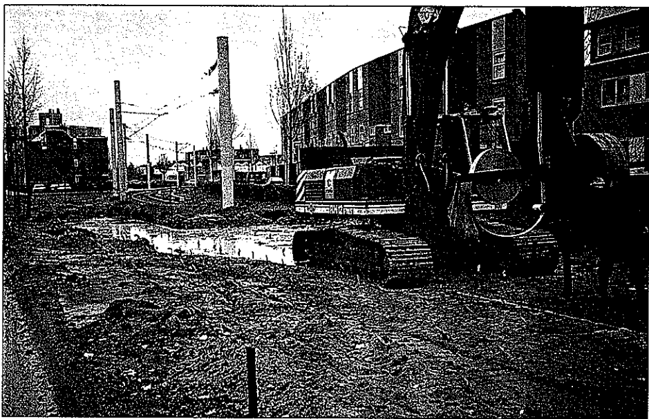
The start of work on the extension from IJsselstein to Zenderpark in November 1998, as piling takes place on the future alignment. C.J. Wansbeek
