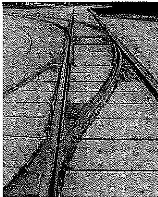
Graphic 4: Picture of Phoenix 37a switch (Source: AVG, Karlsruhe)
