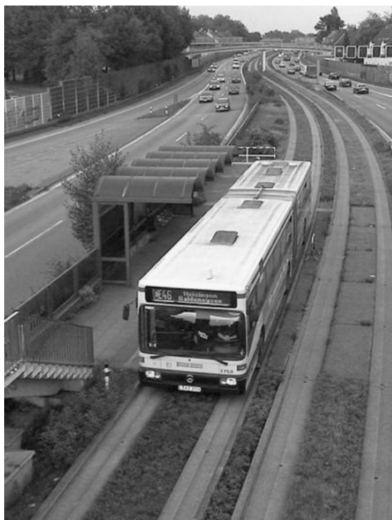
Photo 5.32 Guided busway in freeway median (Essen)
