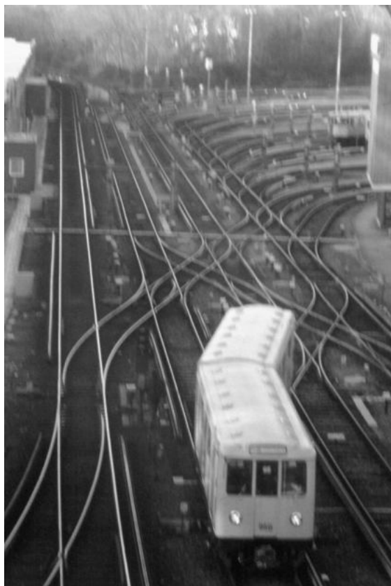
Photo 6.23 Track layout in a rapid transit yard with many types of track switches and crossings on Berlin U-Bahn
