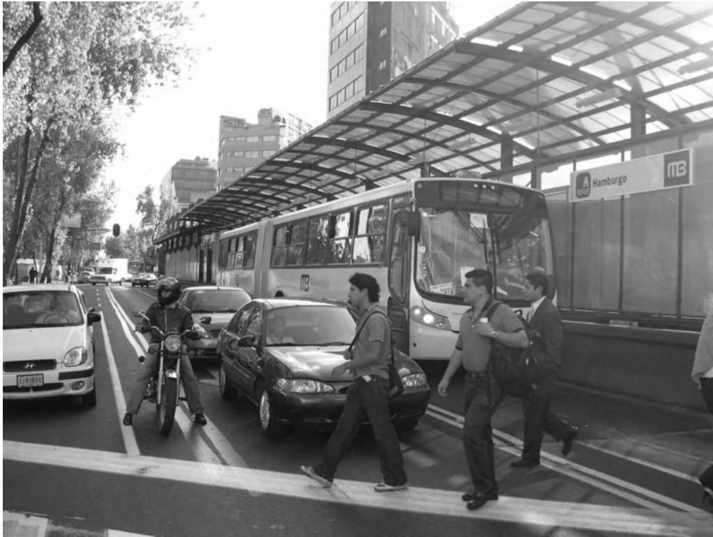
Photo 5.34a BRT Insurgentes Line in Mexico City: high-floor bus at a station (Courtesy of Christopher Puchalsky)
