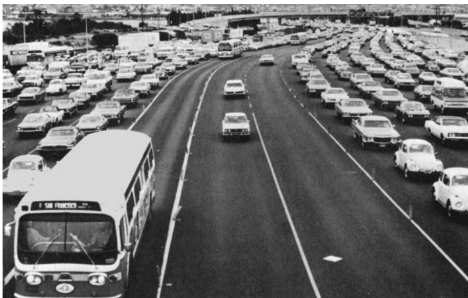
Photo 5.20 Regular bus lanes through the toll plaza area on the San Francisco Bay Bridge. Each bus carries during peaks more persons than all cars which can be seen in two of the adjacent lanes (Courtesy of FHWA/DOT)
