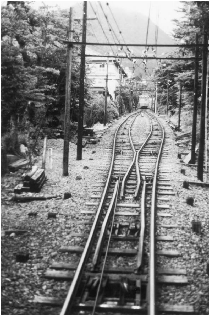
Photo 8.6 Switch and turnout for a single-track funicular (Hakone, Japan)
