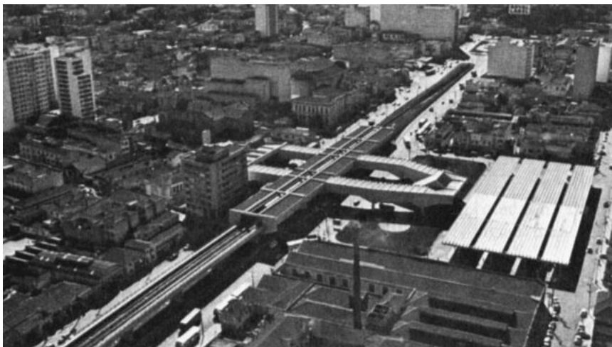
Photo 6.41 Aerial RRT station with direct transfer to bus terminal (São Paulo) (Courtesy of Companhia do Metropolitano de São Paulo)
