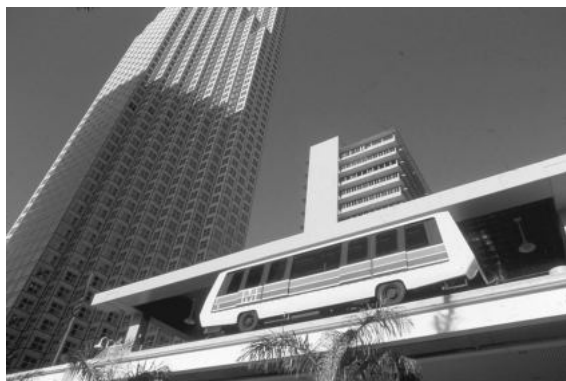
Photo 10.2 Automated guided transit (Miami)
