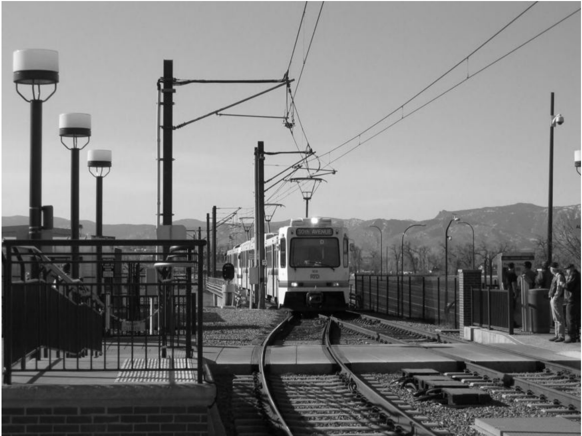
Photo 6.33 LRT stations with simple pedestrian crossings
