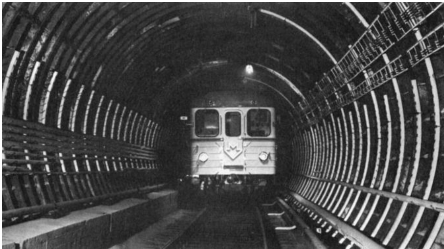
Photo 6.30 Bored tunnel in Prague with Soviet-designed standard RRT vehicle (Courtesy of Praha Metro; photo by Antonin Plevka)
