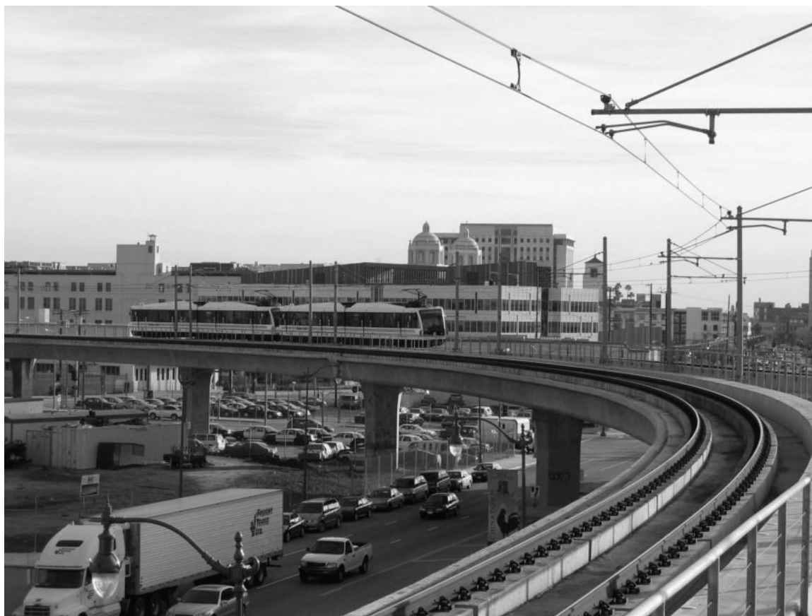
Photo 6.21 Direct-fixation track with rails fastened to the concrete base on Los Angeles LRT Pasadena ("Gold") Line (Courtesy of James Aslaksen)
