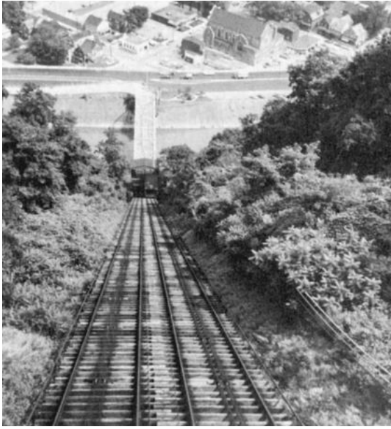
Photo 8.7 Double-track funicular for passengers and automobiles (Johnstown, PA) (Courtesy of Richard Clarke)
