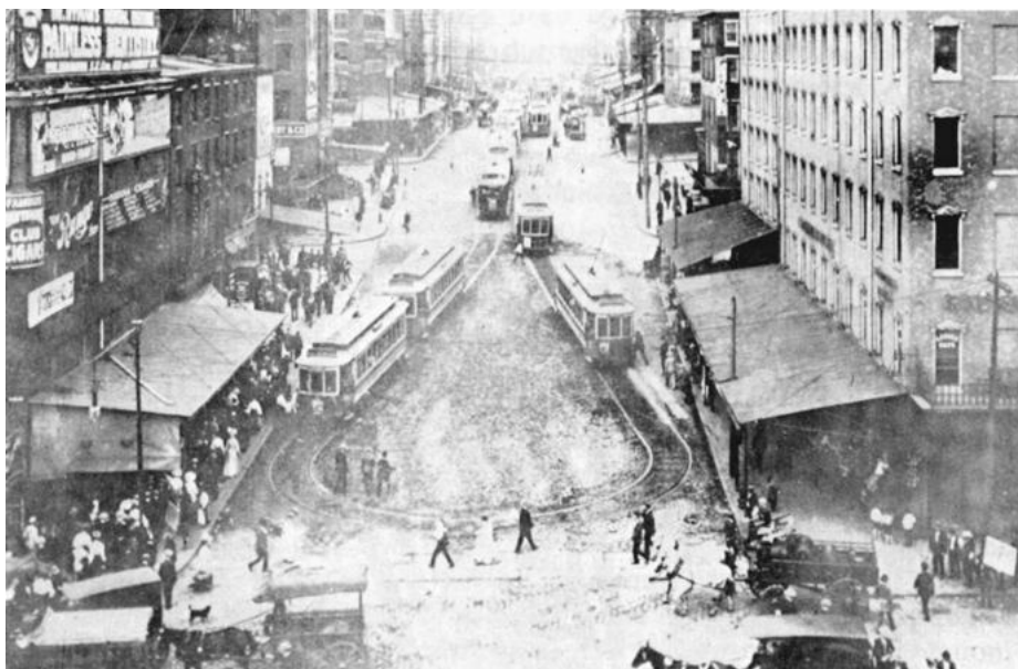
Photo 1.5 Streetcar terminal on Market Street at Delaware Avenue in Philadelphia, 1900
