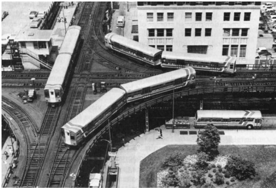
Photo 6.24 Entrance to the Chicago "Loop." Substandard at-grade crossing but handles record train frequencies (Courtesy of CTA)
