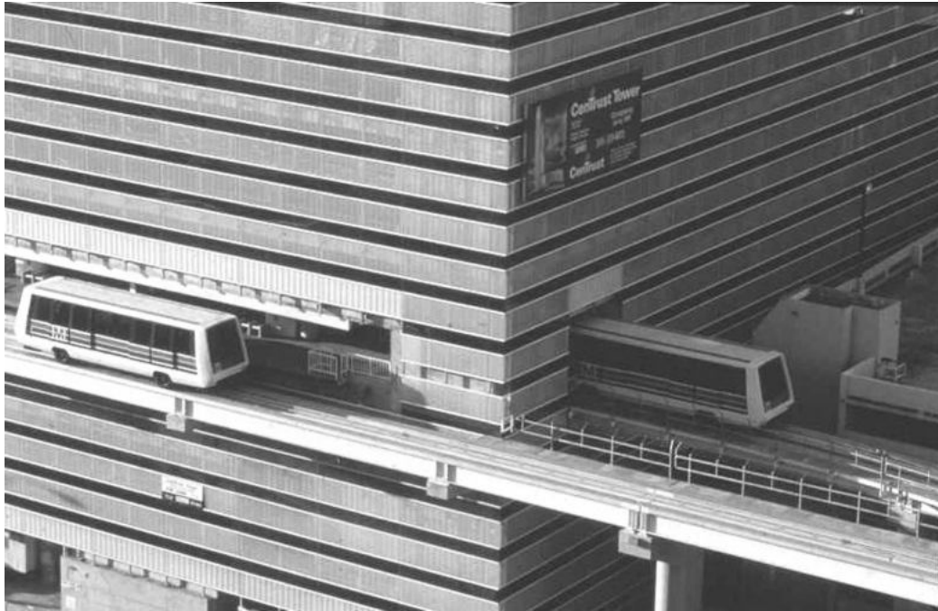
Photo 7.3 Miami DPM guideway penetrates CBD (Courtesy of Westinghouse Electric)
