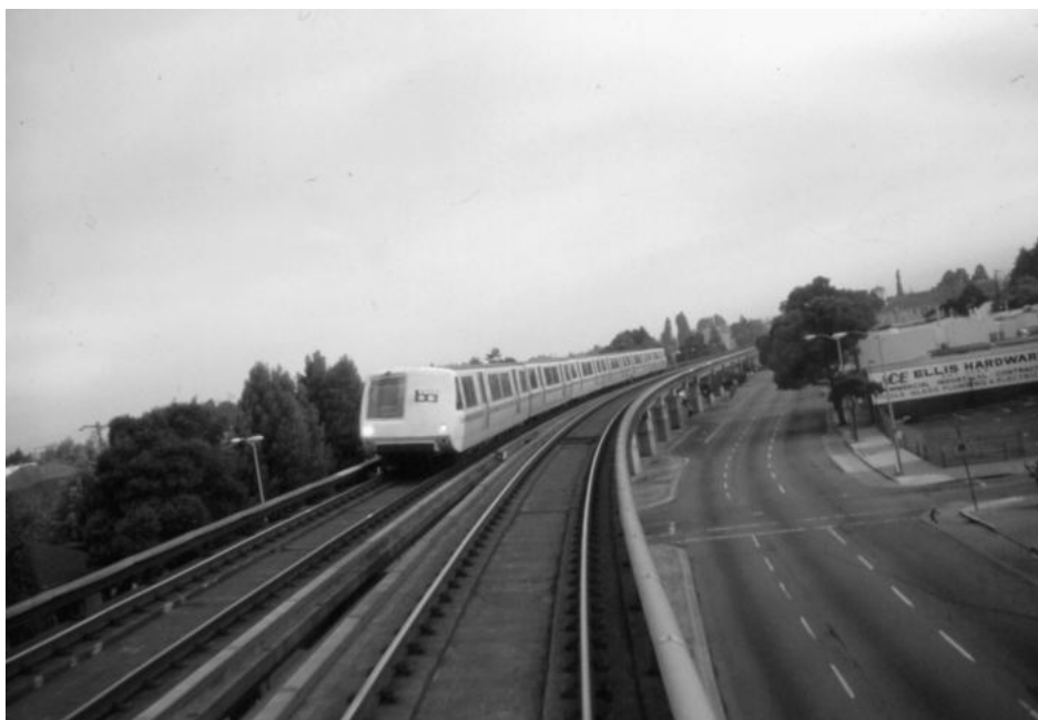
Photo 6.28 BART train on aerial structure
