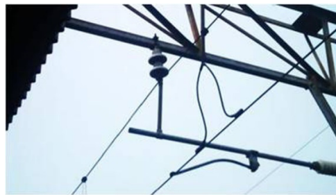
Fig. 2. Simple catenary single trolley wire
